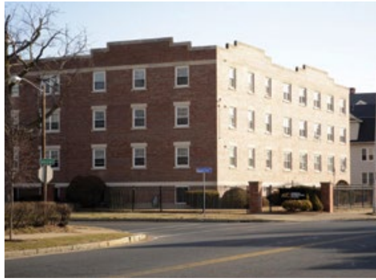
View of Magna Hall from the corner of Northampton Ave.
